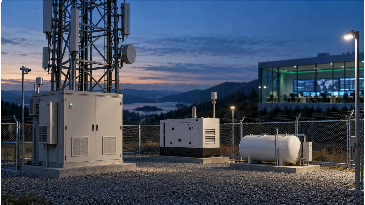
Remote Cell Tower Monitoring: From Site Alarms to Maintenance Action
